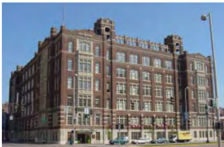
Figure 28: The Emery Center Apartments on Central Parkway.
