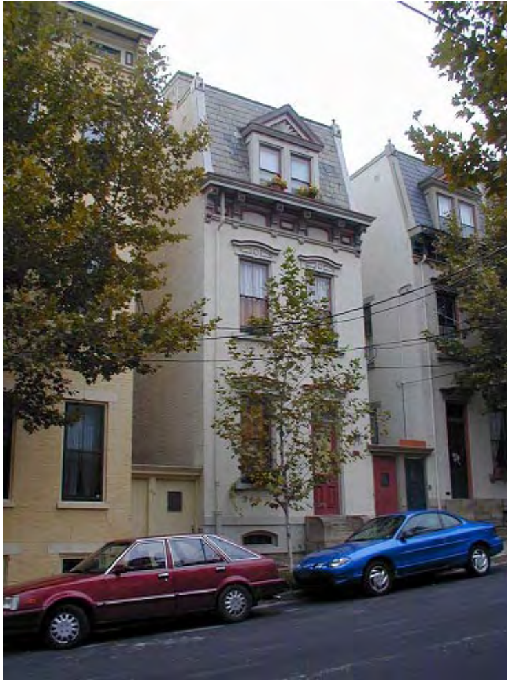
Figure 26: Single family residences on 14th Street.
