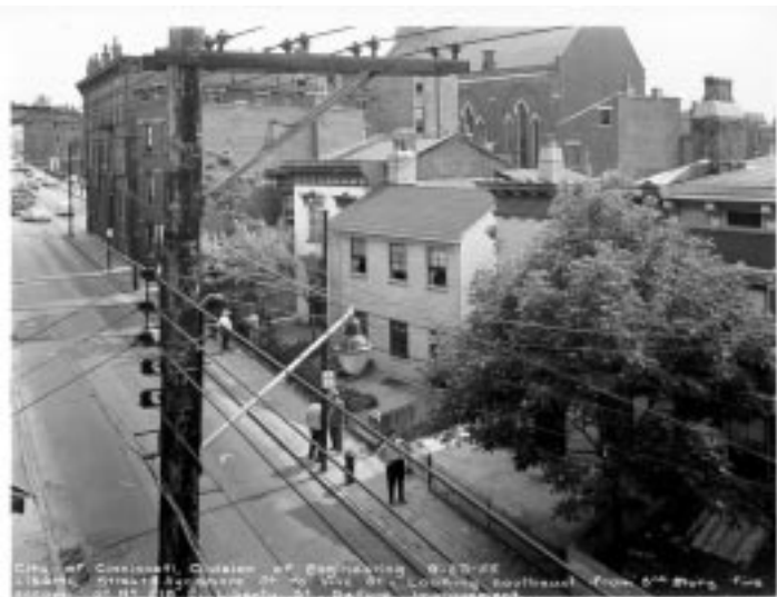
Figure 100: Liberty Street between Sycamore and Vine Streets in 1955 before street widening.
