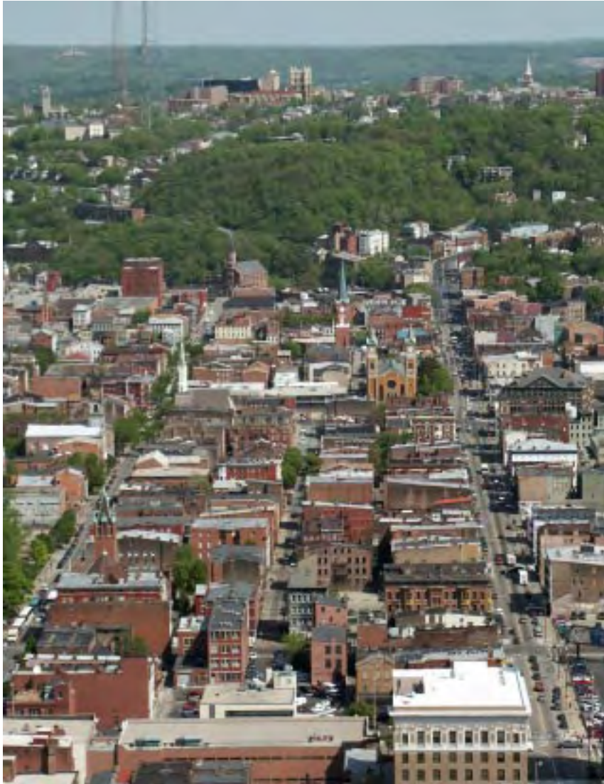
Figure 9: An aerial view of OTR. Photo courtesy of Daniel Young.
