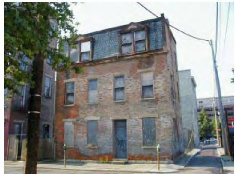
Figure 22: A vacant building on 13th Street
