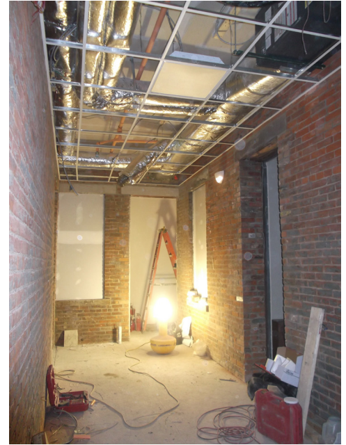
Unfinished interior of an ESSH apartment
