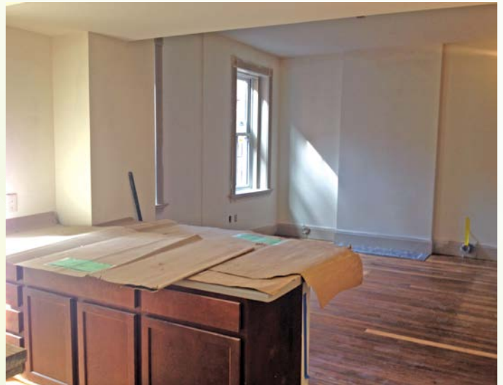
BP Renovation Interior
